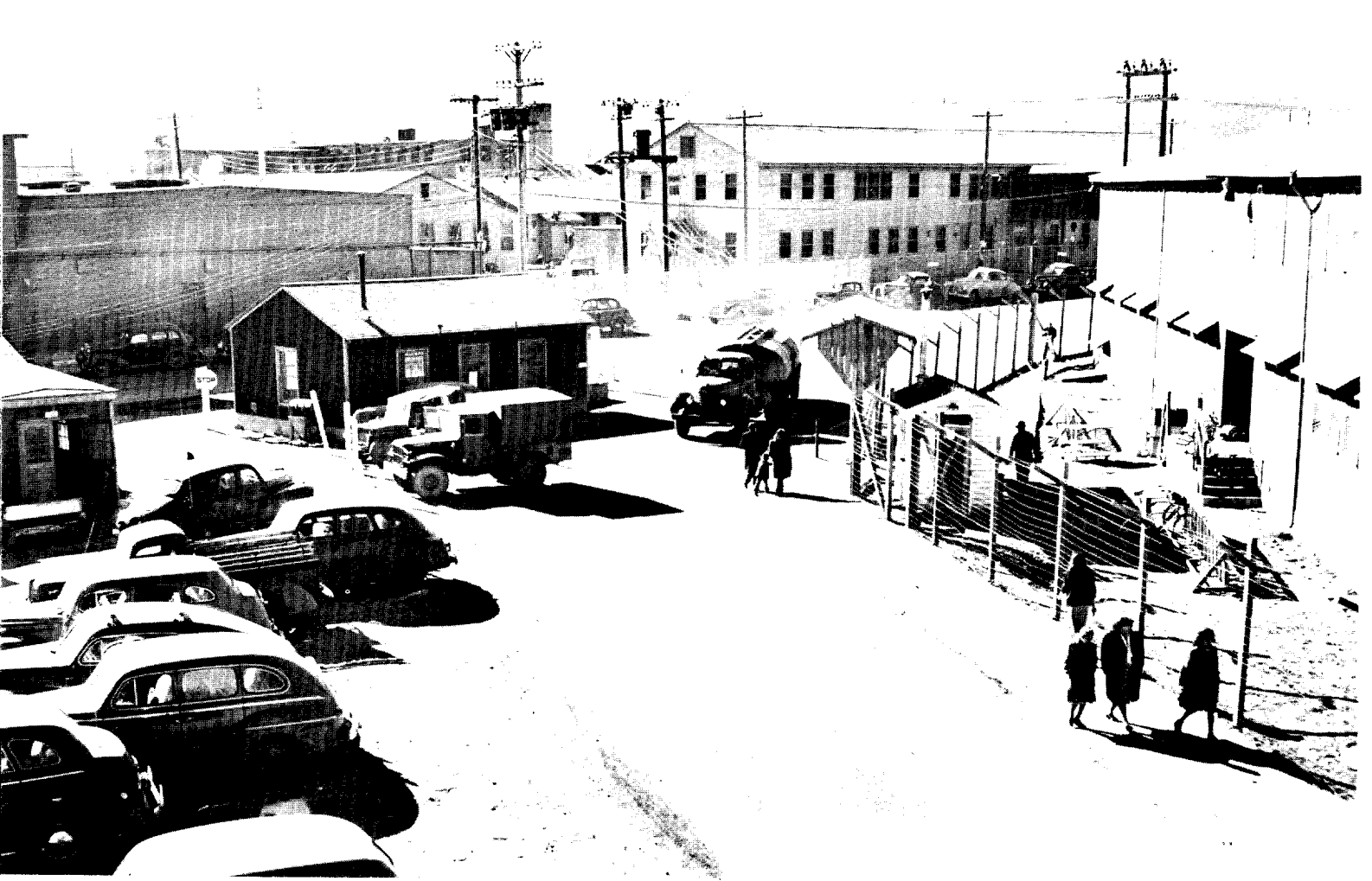
Atomic bomb research was conducted in these hurriedly constructed laboratory buildings which made up the
